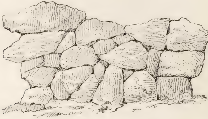
FIG. 62.—Wall on the Bali Dagh.
